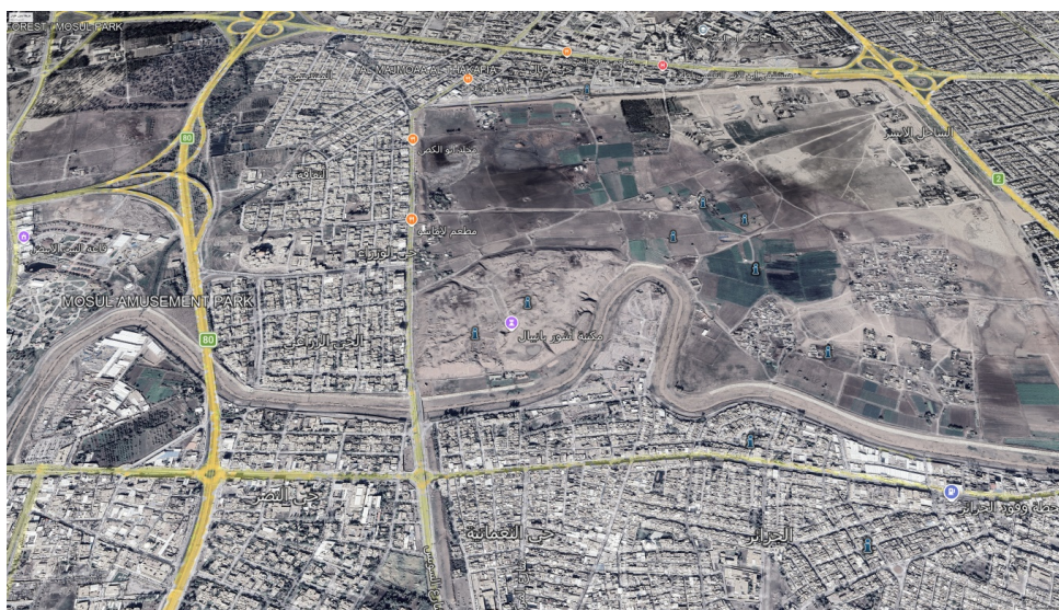
Figure 3. Present-day satellite image showing the Khosr River bending around the southern and eastern vicinity of Tell Kuyunjik within the urban area of Mosul/Nineveh. The view illustrates the close spatial relationship between the river channel and the principal archaeological mound. Source: Google Earth.
